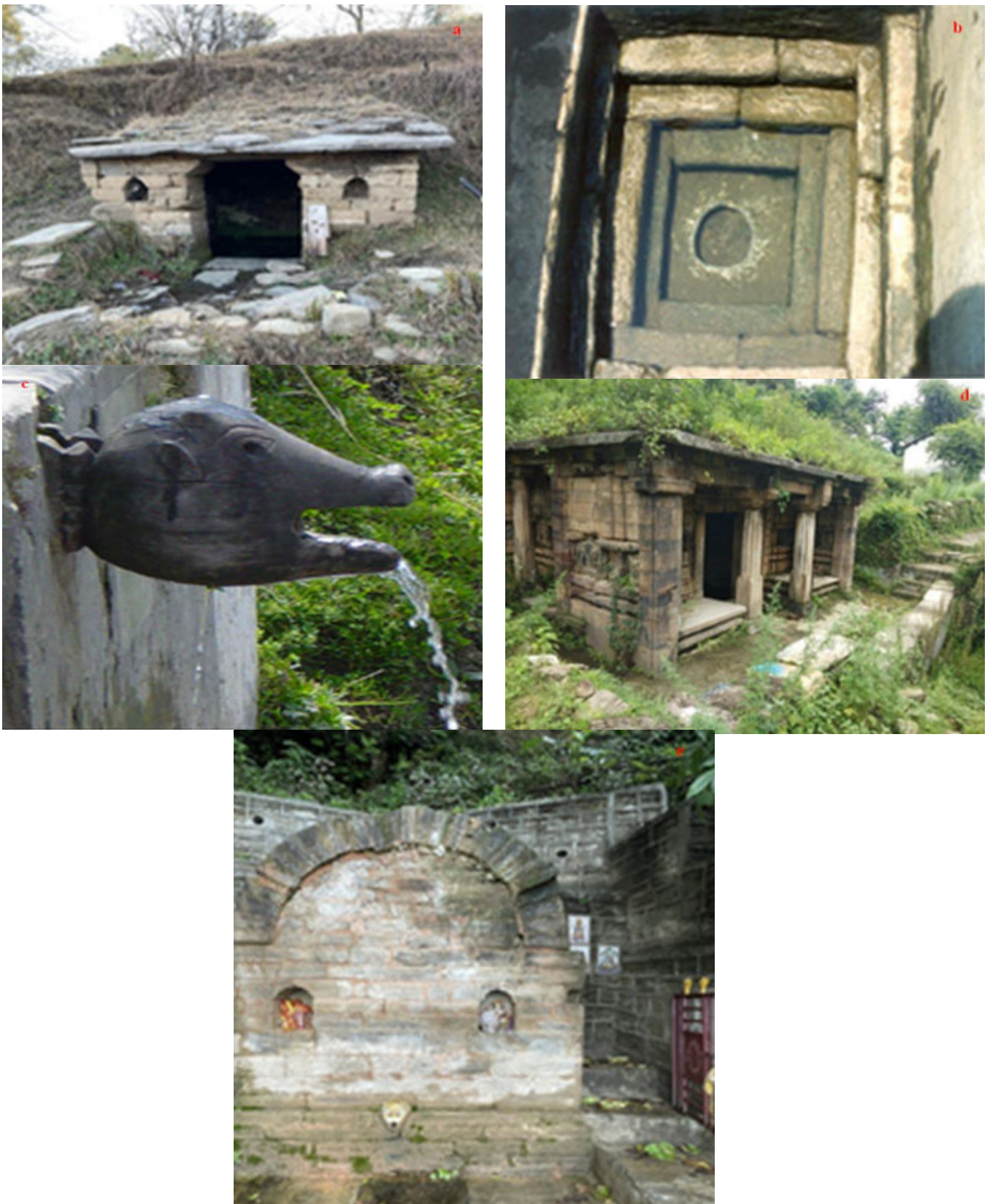
Figure 1. Traditional water sources in Uttarakhand - Naula (a), inner view of Naula (stepwell) with water stored (b), and Dhara (c). Many of these (Naula (d) and Dhara (e)) are now dried and defunct in this region (Photo credits: Deep Bisht, Almora)
